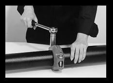
Tighten the nuts alternately, bringing coupling halves together (metal to metal). Then apply specified torque to ensure proper contact between coupling halves. Important: Make sure that the coupling halves make good contact in the grooves.
